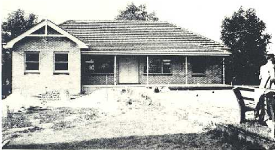
Present club house nearing completion, 1956. Photographer facing north.
